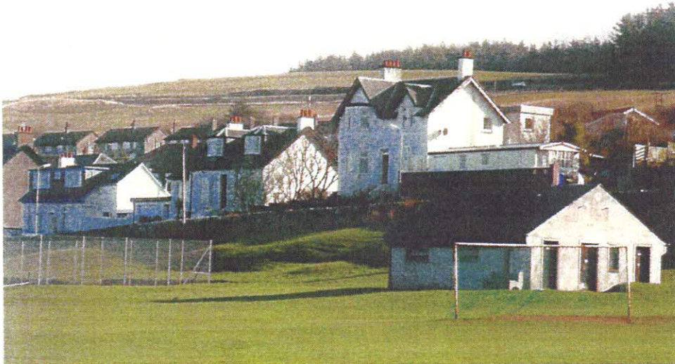
Fig 40: Castle Road showing the two white single-storied houses which comprised "The Roaring Camp". The left hand bungalow (above the tennis court) is the one through which the White Lady referred to earlier on page 23 is reputed to walk
